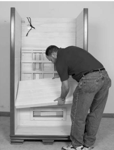
1. Place bottom (Figure 3, page 3) on a solid flat surface with 5 supporting blocks down. Note: Two blocks on the top of the base go towards the back.
